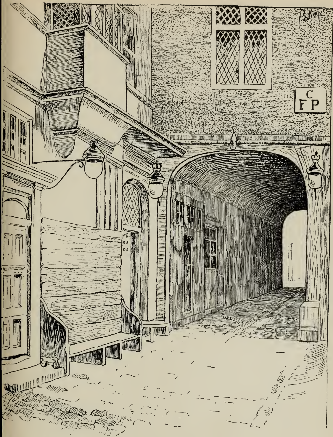
THE ENTRANCE TO SPEAKER'S YARD AS IT APPEARED BEFORE THE FIRE.
